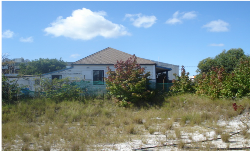
Photo 5 – No. 3 Ewan Street - commercial premises adjoins to the east.
