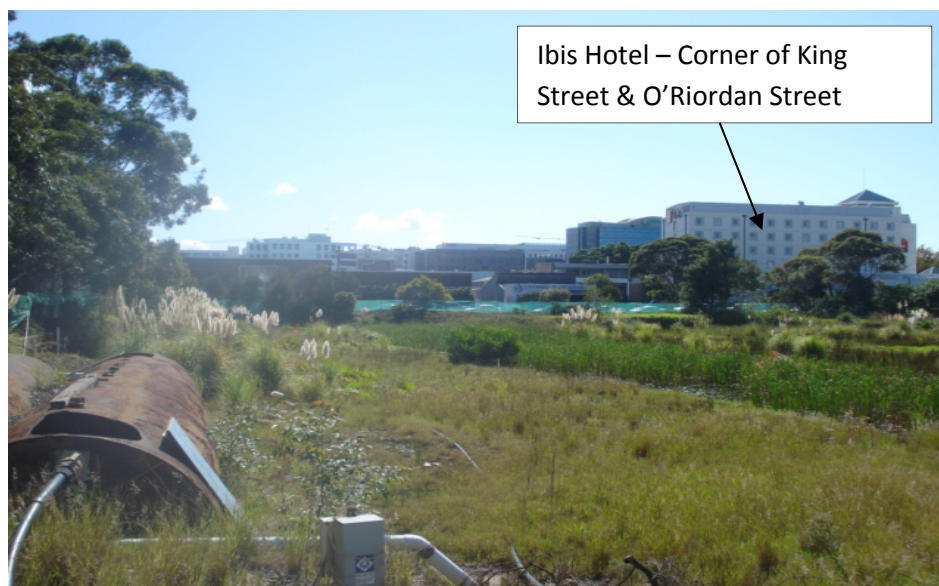
Photo 1 – View of site looking north. Groundwater treatment tanks in foreground.
